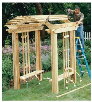
**RIP** 5/4 x 6 cedar decking in half to make the roof lattice. Round the cut edges of each piece with a hand plane. Start in the middle and work each way, spacing the slats 2-5/8 in. apart. Screw them to the arches with 2-1/2 in. screws.
