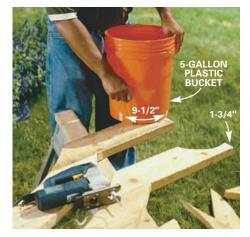
**CUT** the remaining pieces using the Cutting List on p. 39. Trace a curve on the ends of the arch assemblies, the lintels and the seat supports. We used a 9-1/2 in. section of the base of a 5-gallon pail with a radius of 5 in. Cut them out with a jigsaw and smooth the edges with a belt sander.
