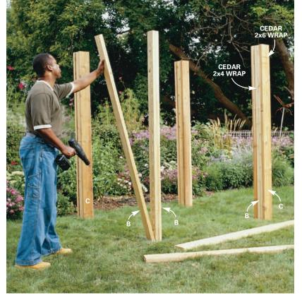
**WRAP** all sides of the pressure-treated 2x4s with cedar. Screw 2x4 cedar on the open sides of the posts and 2x6 on the bench sides of the posts using 3-in. deck screws. Be sure the tops of all the pieces are flush.
