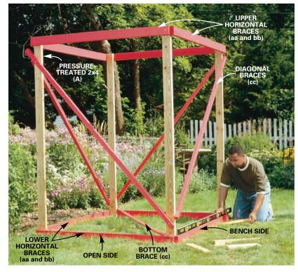
**BUILD** the post framework first, then before you pour concrete into the 18-in. deep postholes, shim and level the assembly. Note: The red lumber pieces are temporary supports to hold the posts in position while you plumb and level and pour the concrete (see text below).
