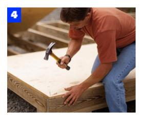
Use 3/4-in. exterior-grade, tongue-and-groove plywood for the floor. Secure the plywood to the frame with 8d nails.
