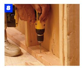
With the wall in position, secure it by screwing down through the bottom 2 x 4 plate and into the floor framing.
