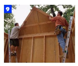
Start the roof by installing the end trusses. Note that the plywood siding is nailed on before the truss is raised. A central 2 x 4 chord stiffens the sheathing.
