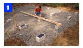
Use a 4-ft. level and a long, straight 2 x 4 to ensure that the concrete foundation blocks are level. Add shims to build up any low blocks.
