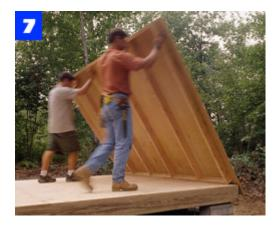
Carefully raise the end wall into position. Note how the plywood siding hangs down to cover the floor framing.
