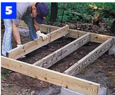
Lay the front and rear joists on the corner blocks. Then, cut the joists, position them
