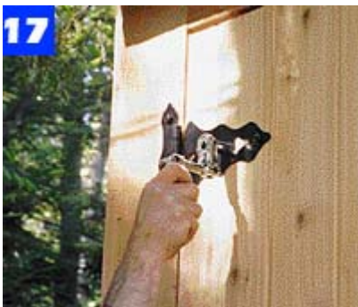
17 Position the door in its opening with a 1/4-in. space at the top and sides. Bore pilot holes for the hinge screws and secure the hinges.
