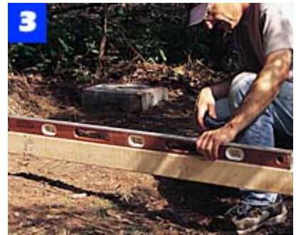
Use a straight 2 x 4 and a 4-ft. level to check that the corner blocks are installed at the same height.
